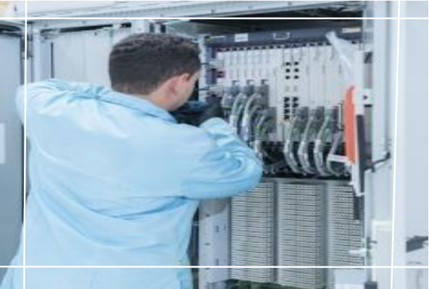
Assembly and installations solution Sorocaba
